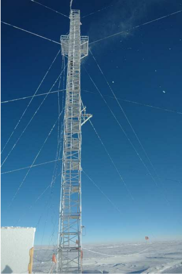
Figure 1. The 45m tower at Dome C. Computers and electronics are located in the shelter at the foot of the tower.
