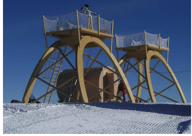
Fig. 1. Concordia astro observatory in November 2004. One can see the two platforms and the wooden igloo between. The DIMM is on the top of one platform.
